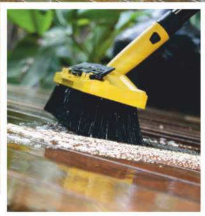
2 Clean the timber Scrub the surface using deck cleaner applied with a stiff-bristled broom.
