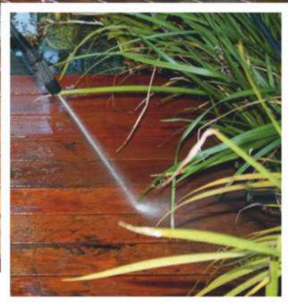
3 Rinse the surface Hose off the deck cleaner and allow to thoroughly dry.
