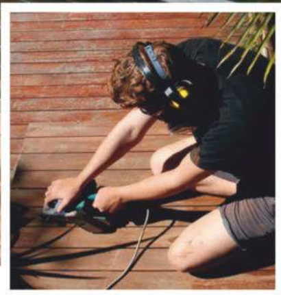
4 Sand rough areas Smooth any rough or marked areas and remove dust. ▶
